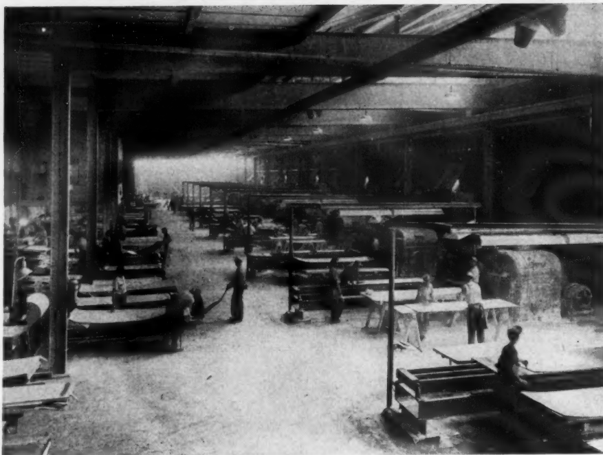
Capacity of the grinding and polishing department, above, of Eastern Stainless Steel Corp., Baltimore, has been greatly expanded as part of the company's over-all modernization program
